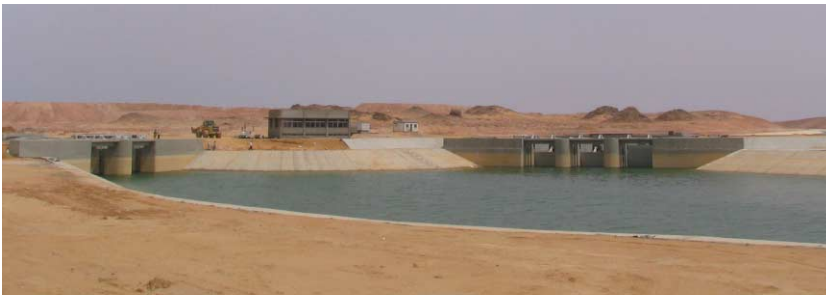
South Valley Development Project (Toshka & East Oweinat, Egypt)
