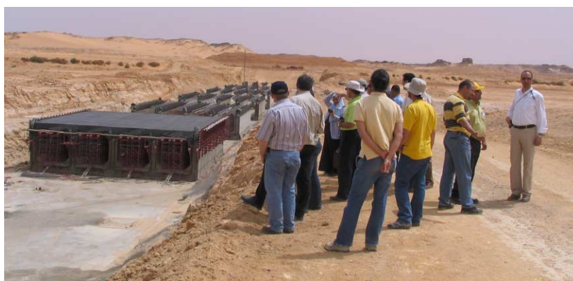
Field trip to the South Valley Development Project: siphon below the Toshka spillway (Egypt)
